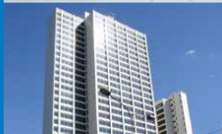
NSSF building , Nairobi (2 x 650 KVA Synchronized)
